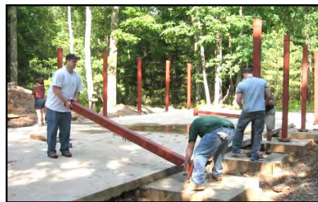
Below: In 2007, roughly 30 construction volunteers and 40 donors replaced the dilapidated staff dining tent with a permanent pavilion, Alumni Hall. Over the course of 3 work weekends and a few days in between the foundations were dug, footings poured, the steel columns and glue lam beams set. The roof was decked, a metal roof installed and the permanent lighting turned on.
