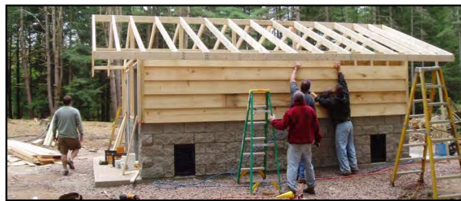
Below: In 2007, roughly 30 construction volunteers and 40 donors replaced the dilapidated staff dining tent with a permanent pavilion, Alumni Hall. Over the course of 3 work weekends and a few days in between the foundations were dug, footings poured, the steel columns and glue lam beams set. The roof was decked, a metal roof installed and the permanent lighting turned on.
