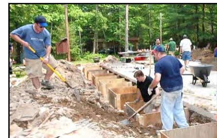
Below: In 2007, roughly 30 construction volunteers and 40 donors replaced the dilapidated staff dining tent with a permanent pavilion, Alumni Hall. Over the course of 3 work weekends and a few days in between the foundations were dug, footings poured, the steel columns and glue lam beams set. The roof was decked, a metal roof installed and the permanent lighting turned on.
