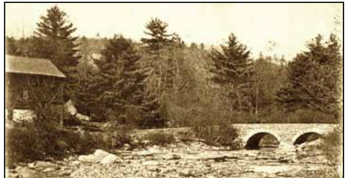
TMR Sawmill & Tusten Stone Arch Bridge
